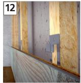
Nails can be used for mounting, using a pneumatic nail tacker or hammer. The 3D profile claws can also be screw-mounted to the substrate. This process applies to the entire wall-mounting. When assembling a ceiling, the profile claws are screw-fastened to the sub-construction.
